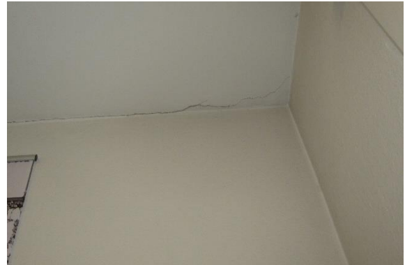
Abb. 66 Riss in Decke
