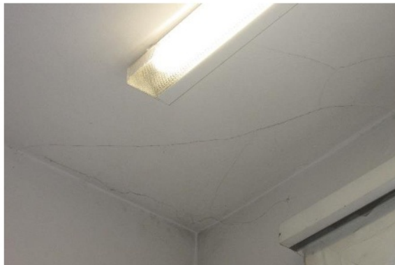
Abb. 43 Riss in Deckenecke
